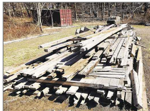
Wood from the 19th-century barn will be used in the new structure. The barn was dismantled and its pieces cataloged so it could be rebuilt.
